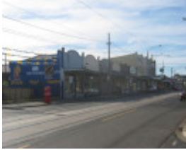
519 -541 Plenty Road, Shops
