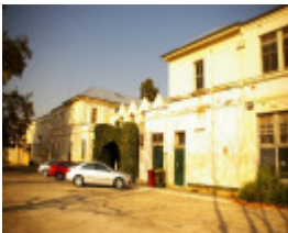
H2170 St Vincent de Paul Boys Orphanage rear Cecil St buildings inc grotto detention plate
