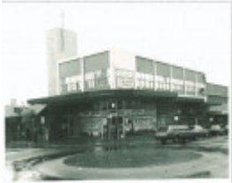
27226 Colonial Mutual Life Building
