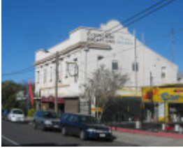
UFS Dispensary (fmr), 2 Gooch Street, Thornbury
