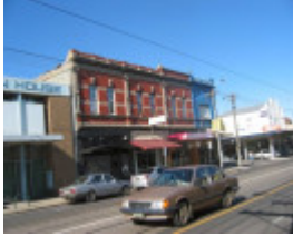
Shop Row 804-810 High Street
