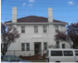
662 High Street, Reservoir
