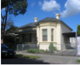
9 Station Street, Reservoir
