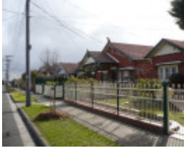
QUEEN ST NTH SIDE LOOKING WEST
