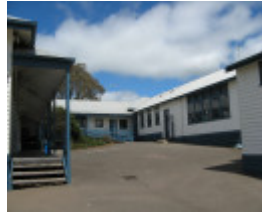
Leongatha Secondary College_rear of 1934 building_Kj_24/10/07
