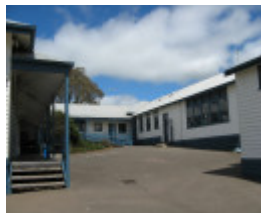
Leongatha Secondary College_rear of 1934 building_Kj_24/10/07
