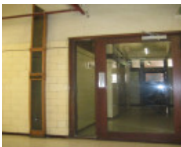
Nicholas Building_Melbourne_Letter Chute_3 Feb 2007_mz
