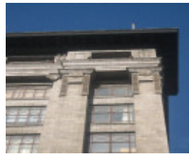
Nicholas Building_Melbourne_Front Facade Detail_13 Feb 2007_mz
