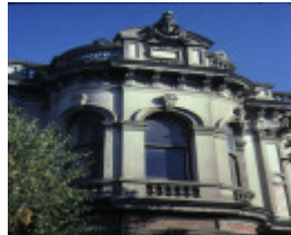
labassa caulfield external windows
