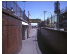
caulfield railway station normanby road caufield underpass nov1984
