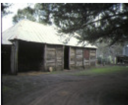
glenisl homestead glenisl via cavendish outbuilding jul1978
