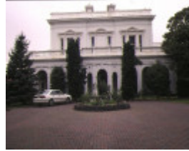
1 tara berwick street camberwell front view
