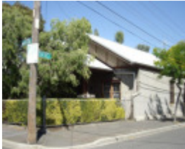
HO34 (1) - House, 24 Buninyong Street, Yarraville.JPG
