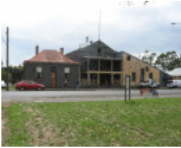
Piper Street view of the complex March 2010
