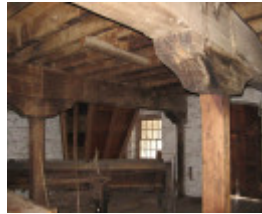
Mill interior Aug 2009
