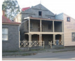
Former Willis Flour Mill Kyneton July 2008 mz Mill
