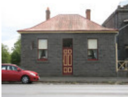
Street facade of residence March 2010
