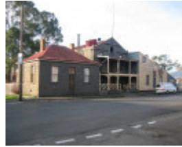
Former Willis Flour Mill Kyneton July 2008 mz Front Elevation
