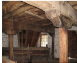
Mill interior Aug 2009
