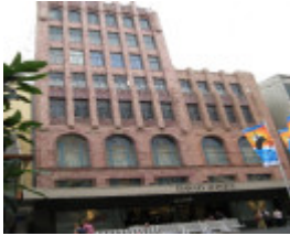
DJs former Coles_front facade_16 Jan 08
