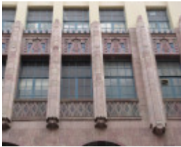
DJs former Coles_rear facade detail_16 Jan 08
