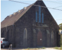
HO63 - Bluestone Church Hall, 30a Pickett Street, Footscray.JPG
