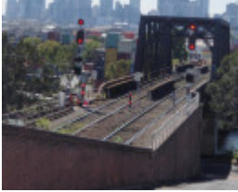
HO107(1) - Rail Bridge over Maribyrnong River & Tunnel, Bunbury Street, Footscray.JPG
