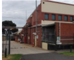
HO113 - Klipspringer 40-54 Cranwell Street, Braybrook.JPG
