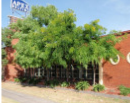
HO129 (1) - Hopkins Odlum, 268 Geelong Road, West Footscray.JPG
