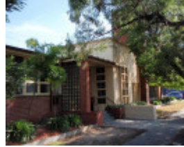
HO129 (2) - Hopkins Odlum, 268 Geelong Road, West Footscray.JPG
