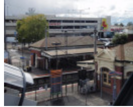
HO49(2) - Footscray Railway Station.JPG
