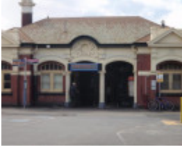
HO49(1) - Footscray Railway Station.JPG
