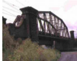
HO51(2) - Footscray Rail Bridge.jpg
