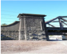
HO51(1) - Footscray Rail Bridge.jpg
