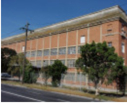
HO 160 (1) - Australian Estate Wool Store, 27-61 Sunshine Road, West Footscray.JPG
