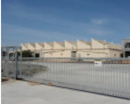
HO162 (1) - Olex Cables, 207 Sunshine Road, Tottenham.JPG
