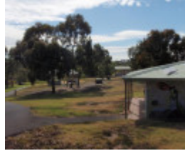
HO64(2) - Former Melbourne Meat Preserving Co. Pipemakers Park, Maribyrnong.JPG
