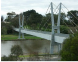
Macintyre Bridge Over Barwon River
