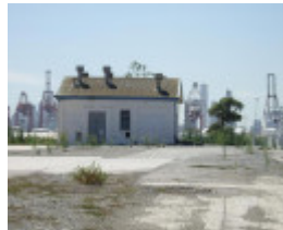
HO179 (3) - Cuming Smith, 221A Whitehall Street, Yarraville.JPG
