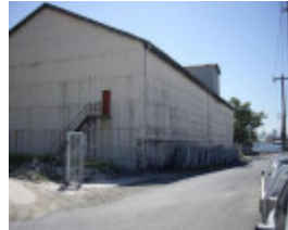
HO75 (2) - Colonial Sugar Refinery complex, 265 Whitehall Street, Yarraville.JPG
