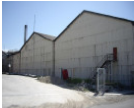
HO75 (1) - Colonial Sugar Refinery complex, 265 Whitehall Street, Yarraville.JPG
