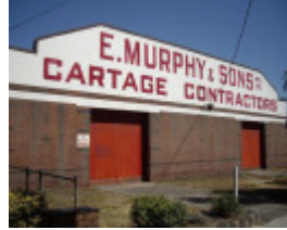
HO182 (2) - Murphy's Transport, 248 Whitehall Street, Yarraville.JPG
