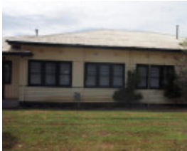
HO135(1) - Pyrotechnic Division 61-71 Hampstead Road, Maidstone.JPG
