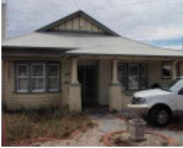
HO141 - Williamson House, 182 Mitchell Street, Maidstone.JPG
