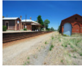
CHILTERN RAILWAY STATION AND GOODS SHED SOHE 2008
