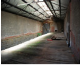
CHILTERN RAILWAY STATION AND GOODS SHED SOHE 2008
