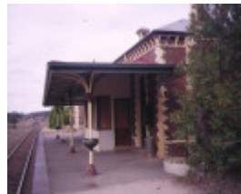
chiltern railway station & goods shed railway avenue chiltern platform verandah apr1995
