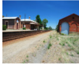
CHILTERN RAILWAY STATION AND GOODS SHED SOHE 2008
