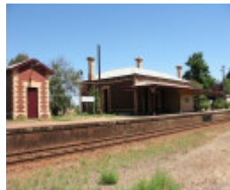
Chiltern railway station Building B1 & Lamp Room B2 February 2002
