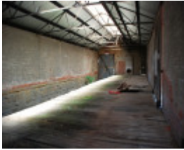
CHILTERN RAILWAY STATION AND GOODS SHED SOHE 2008
