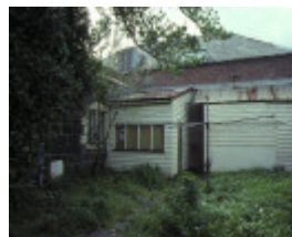
Barwon Bank Riversdale Rd Marnock Vale Newtown Kitchen Wing Sep 1977
