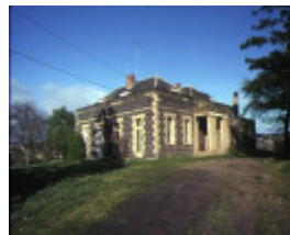
Barwon Park Riversdale Rd Marnock Vale Newtown Front View Sep 1977
