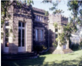
h00425 1 barwon bank riversdale road marnock vale newtown south west cnr she project 2004
