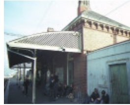
clifton hill railway station complex hoddle street clifton hill side view jun1984
