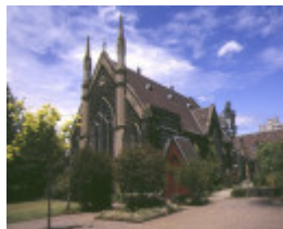
1 former independent church malvern road armadale west elevation feb1994
