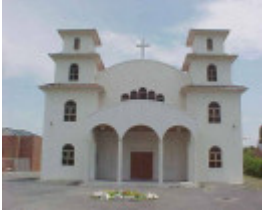
View from Amis Crescent
