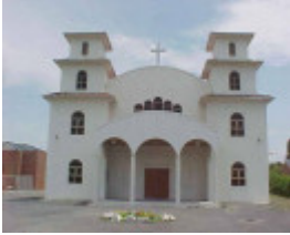
View from Amis Crescent
