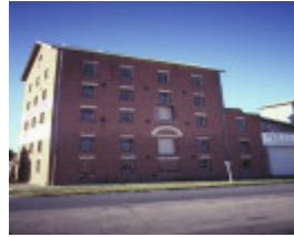
1 echuca flour mill side view of mill
