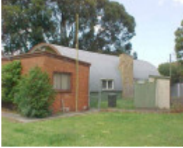
View of building from north-west
