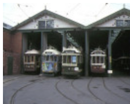
1 bendigo tram sheds front view of tram sheds
