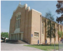
Church (1959) viewed from south-east
