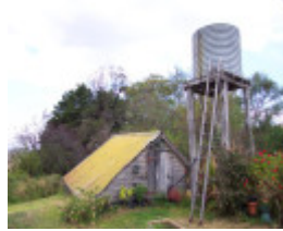
Underground water tank with gable roof and header tank
