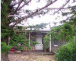
Glencoe (prior to renovation)
