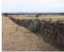
Dry Stone Wall R300
