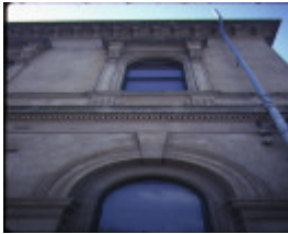
clunes post office detail exterior windows nov1984
