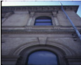
clunes post office detail exterior windows nov1984
