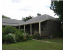
Correagh former kitchen wing
