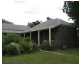
Correagh former kitchen wing
