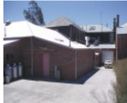
club hotel clunes rear view feb1991
