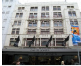
David Jones_1911 building & 1925 addition_16 Jan 08
