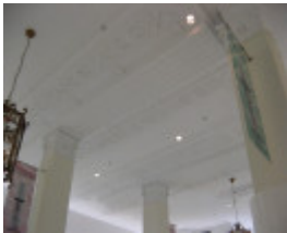
David Jones_plaster ceiling_16 Jan 08
