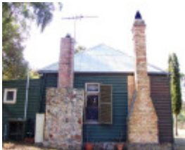
Paine's Cottage Chimneys
