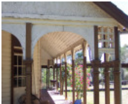
Cornwall Park Stud - verandah detail
