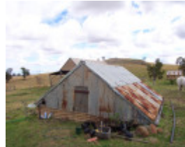
Underground water tank
